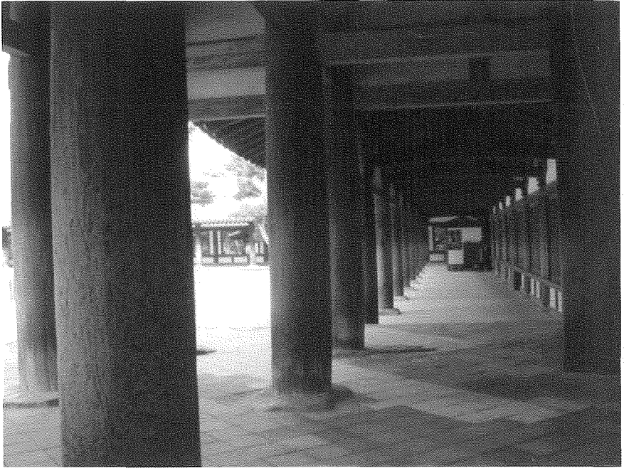
FIGURE 11.1 Columns with entasis, Hōryū-ji Temple. PHOTOGRAPHED BY THE AUTHOR.
